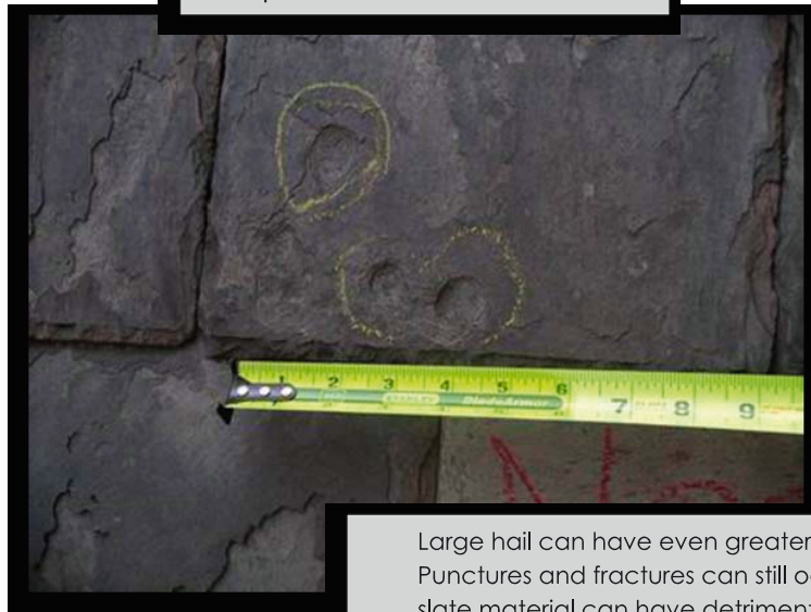
Compression marks in S-2 Slate
