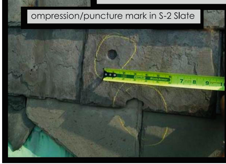
The s-2 Grade Pennsylvania slates which cover this roof slope have been pelted with hailstones leaving both impact punctures and compression marks. There have been newer S-1 Grade slates installed during maintenance and repairs.
