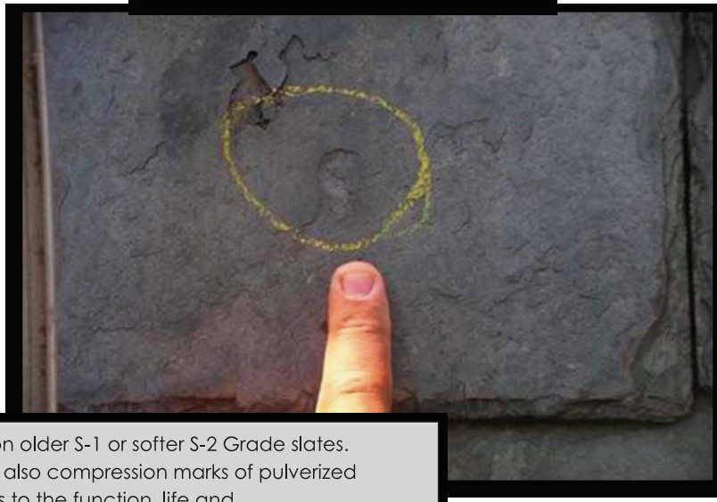
Compression mark in S-2 Slate
