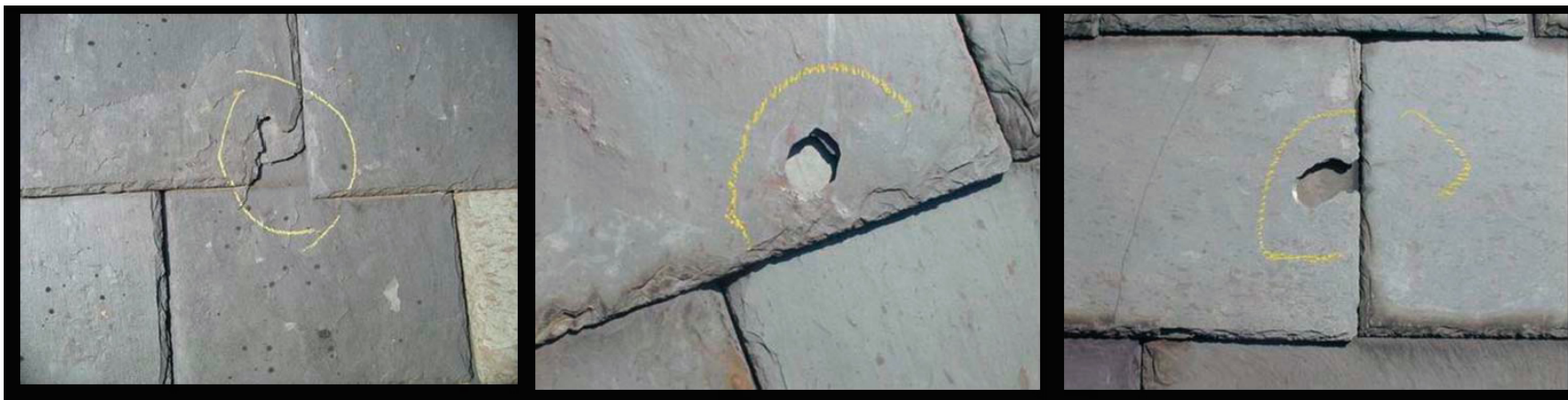
Compression marks in S-2 Slate
